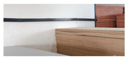
Fig. 270: Safe Stacking Height (max 3-4 feet)
