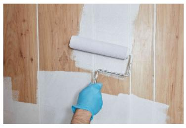
Fig. 41: Paint over wood paneling
